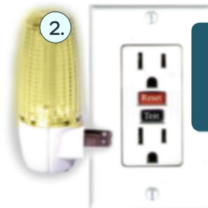
Plug in an ordinary night-light into the GFCI and turn it on. The light should now be ON.
